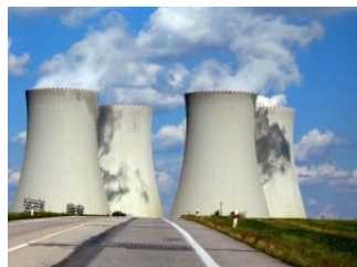
Cooling Towers https://whatistreatment.wordpress.com/what-are-the-systems-associated-with-water-treatment-and-how-are-they-treated/103-2/
